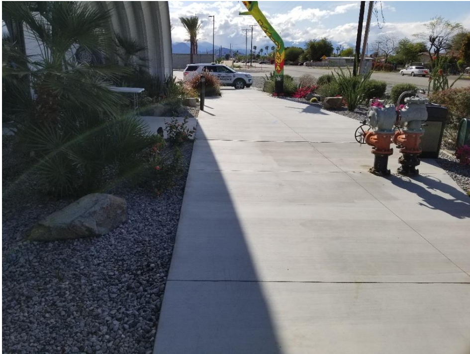
Front Entry is missing “Bicycle Racks”
